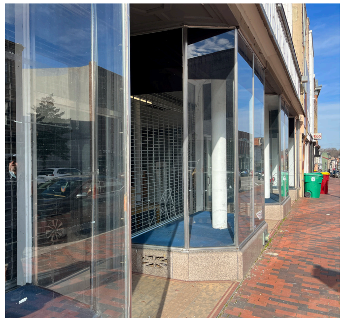
Existing empty storefront window well suited for artwork
